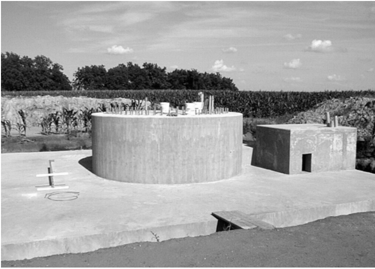
Figure 7. Inverted “T” Slab Foundation
